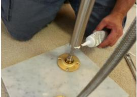
Lower Stands over the flex water supplies. Add caulk or Lock Tight to threads and screw stands all the way down !
