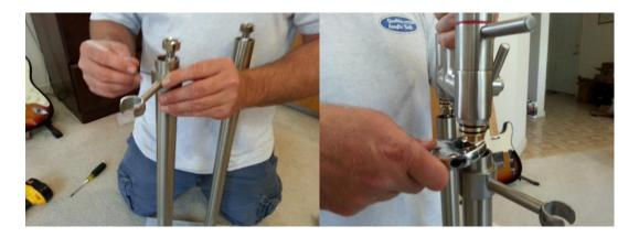
We try to install the faucet adapter (Brass connection between the faucet and stand) IF we forget, Please use 7 wraps of gas pipe teflon tape in yellow and pipe dope on the top going into the faucet
